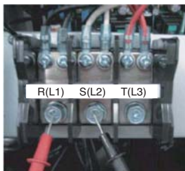
* Measuring input voltage
